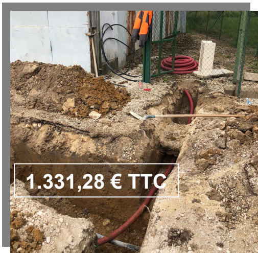
TRAVAUX RACCORDEMENT ENEDIS BAT TECHNIQUE
